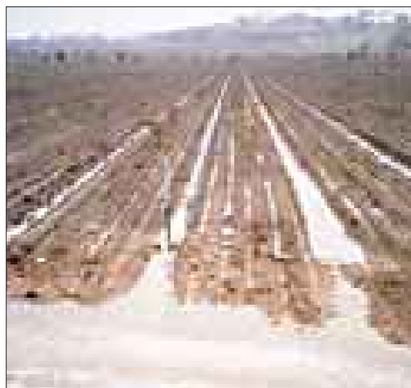
Figure 10. View of water flowing from furrows and the quantity of flow in the Catch Drain (foreground). This runoff occurred at Woodanilling in early July 2000 from an intense storm of about 20 minutes duration. The length of furrow is about 300 m and the slope is about 1.5%.
