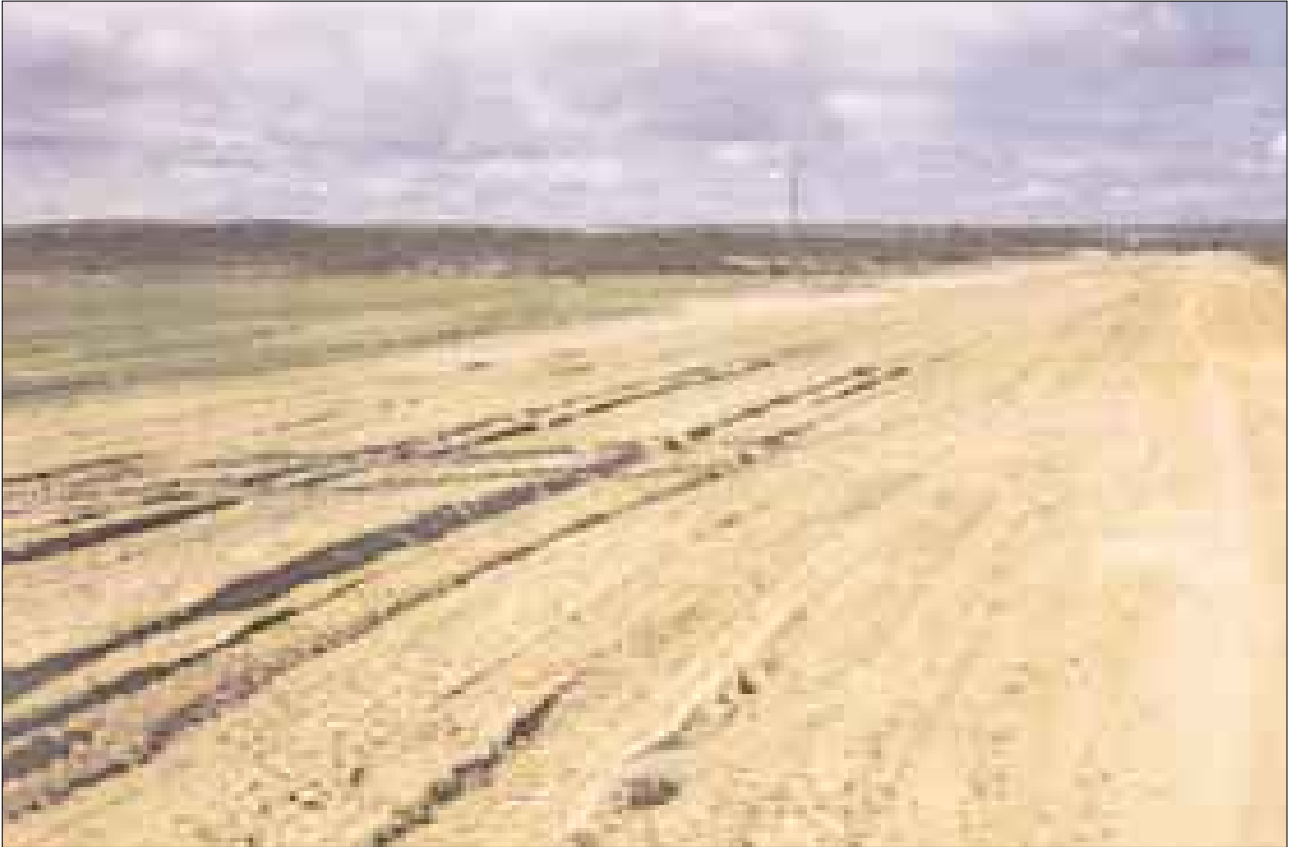
Figure 12. A broad channel of a main Catch Drain and a broad-based bank suitable for turning large machinery comfortably without damaging the channel floor, at Badgingarra.
