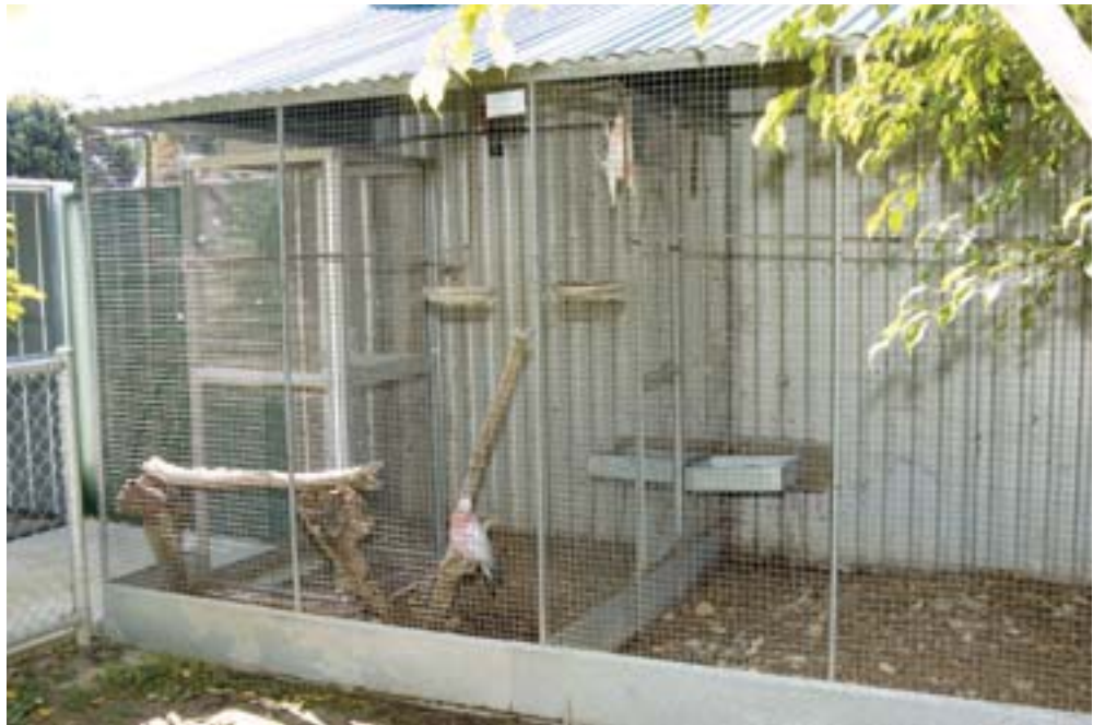
Aviary showing double door, covered roof and some rodent proofing
