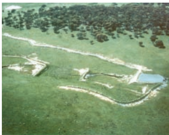
Using a combination of systems, such as drains, banks, roaded catchments and dams, is likely to produce the best results when trying to manage surface water and near surface recharge.
