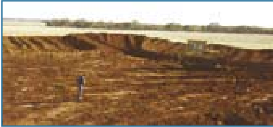
First floor exposed and ready for ripping.
