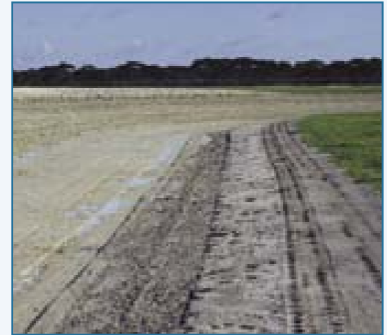
Half-road at Lake Grace used to improve water capture and improve reliability of farm dams.
