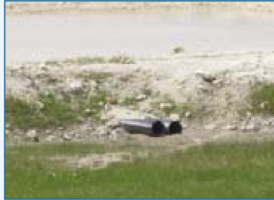
Farm dam with a wing bank and inlet pipes.
