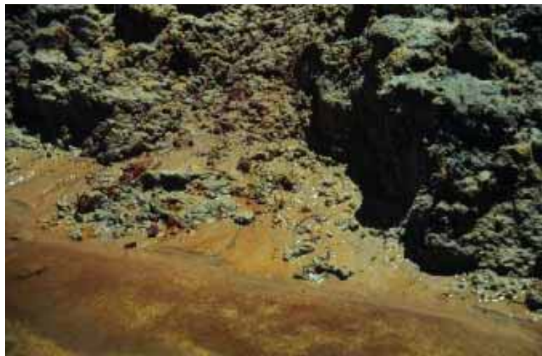
Photo 2: One of the few major seepage zones. Note: the collapse of material at the seepage zone which is in the centre of the photograph.
