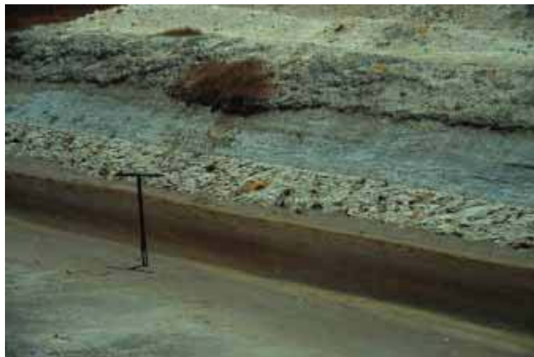
Photo 3: With the exception of a few sites, the soil profile along the main drain is very tight silty clay. Note: The bed of the drain is filled with silt.
