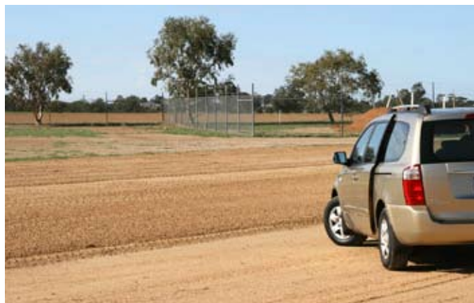
The wide shallow channel enables water to reach the dam without impeding vehicles on the field day site
